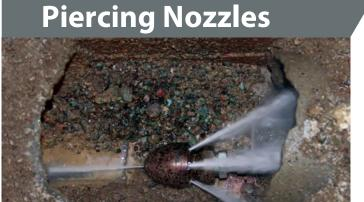
Tiny stones and soft tree roots with some wastes sometimes block the water flow route partially; one of the most practical solutions for clearance without damage is using Piercing nozzle.
